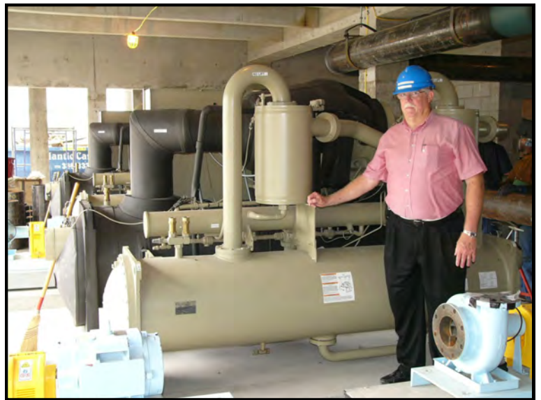
Above photo, Rand is standing next to one of the three Trane 300 ton chillers in the services room.
