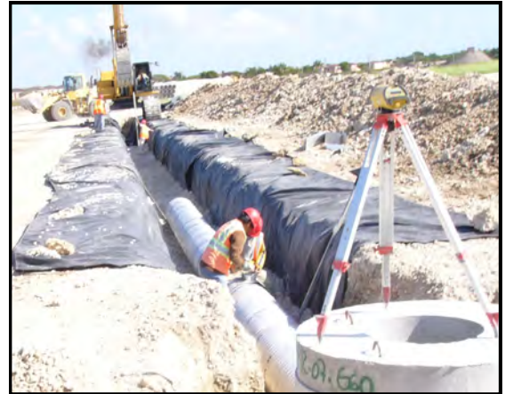
(Above) Two Redland employees join 30' long corrugated aluminized steel pipes from Metal Culverts, Inc. Redland prefers the steel pipe over HDPE plastic pipe because of the ease of installation.
