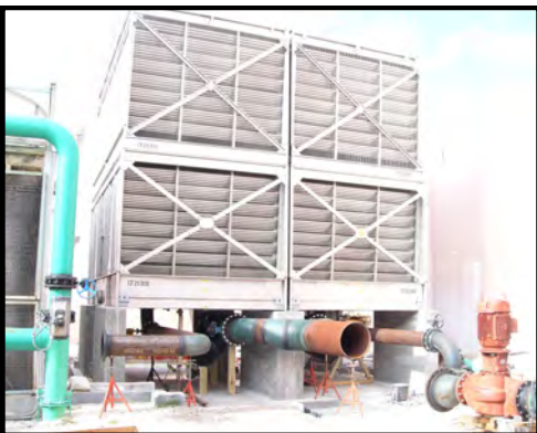
The photo (to right) shows two cooling towers, ready for installation, in the parking lot behind the Hospital. The photo (on left) is of two other towers that are in place and ready for connection.
