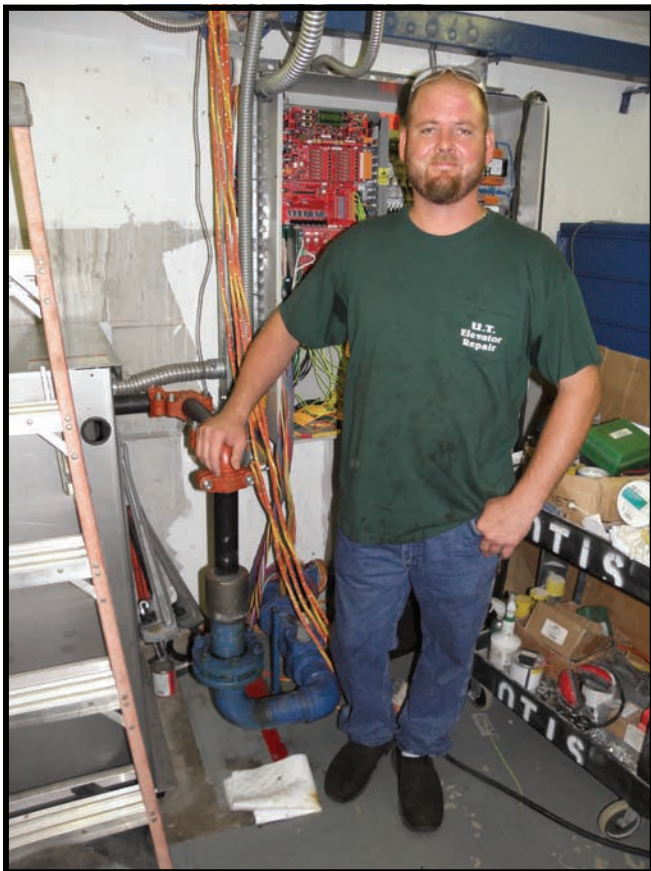
Below- A new piston is installed within the cylinder. Other new parts- tanks, valves, pumps, fluid reservoirs, controls, and piping.
