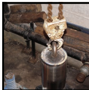
Below- A new piston is installed within the cylinder. Other new parts- tanks, valves, pumps, fluid reservoirs, controls, and piping.
